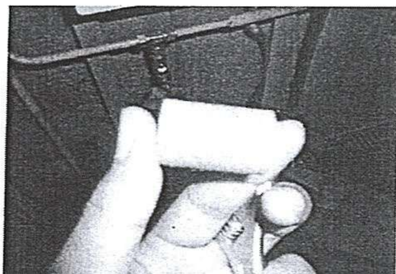
Cleaned filter air purge for HCL stack1,stack2
